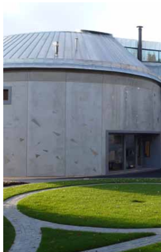
Above: The building comprises 56 irregular precast panels Below: Temporary jambs were cast in the window openings to ensure the structural integrity of the panels
