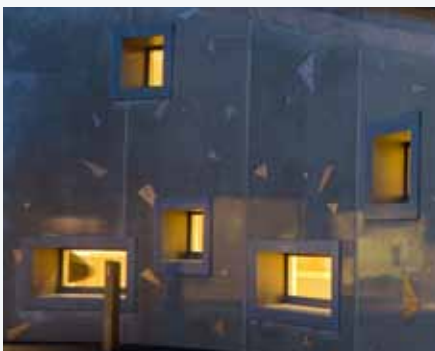
Above: The building comprises 56 irregular precast panels Below: Temporary jambs were cast in the window openings to ensure the structural integrity of the panels
